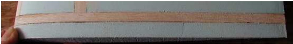
**PRE-BAGGING .003 GLASS TAPE TO LE'S:** Prop up panel. Cut pieces 3" over length. Stick up vertically with masking tape at the ends. Make 2-3 passes with 3M77. Let dry a minute. Stick clean masking tape over the sprayed ones to handle. Starting at an overcap, center the tape.
