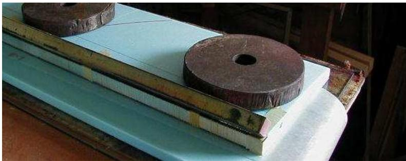
Separately first attach shimmed spar to core rears. Use masking tape & weights to keep it flush to core & beds so no wrapped spar protrudes above the core. Any bottom oozing will be flattened to the wax paper & not interfere with later spackling there.
