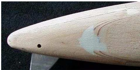
Here a solid bass nose block is shown. The 1/8" balsa doubler has been feathered into the 1/16" SS during sanding to shape. The fill is Icing putty mentioned in the Fine Finishing file. The longer the nose, the further the fill will extend forward.
