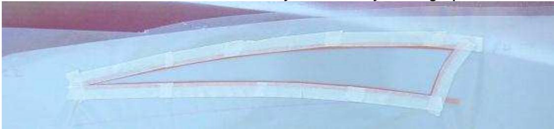
After the first swoosh was painted (see orange in pic below) that masking was removed and with that paint well dried, overall masking for the white second swoosh was applied. Masking must be quickly removed before paint edges dry and stick to it. Tabs are put on all tapes to easily grab and pull.
