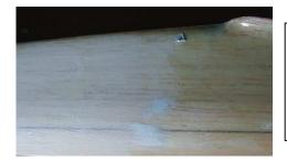
Left area shows the cloth brushed on with resin & block sanded dry with #80 grit. On the right the resin has not yet been sanded. All the shine is to be removed so the next coat will stick.
